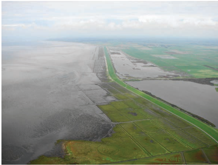
Figure 4.1: Dike built in 1980/81 at the Danish-German border of the Wadden Sea to shorten and strengthen the line of defence. The embanked area is maintained as a semi-natural wetland. In front of the dike, a foreland has been developed to dissipate wave energy. Further off the dike, natural saltmarsh succession has commenced (lower left), (Photo: K. Reise).
