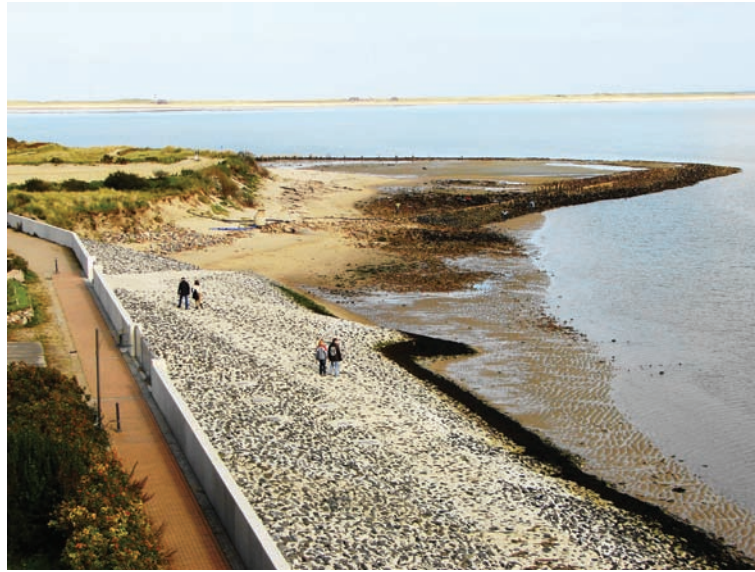
Figure 4.2: While exposed beaches at Sylt are regularly replenished with sand nourishments to combat erosion, its more sheltered Wadden shores are still enforced with new hard structures. More sustainable in the face of sea level rise would be dunes and beaches created with sand borrowed from the North Sea (Photo: K. Reise).
