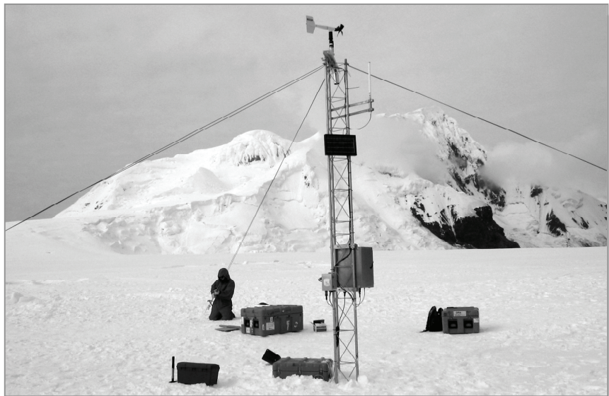
Fig. 16.1: Installed tower on Peter I Island with the peak of the island in the background (looking south)
