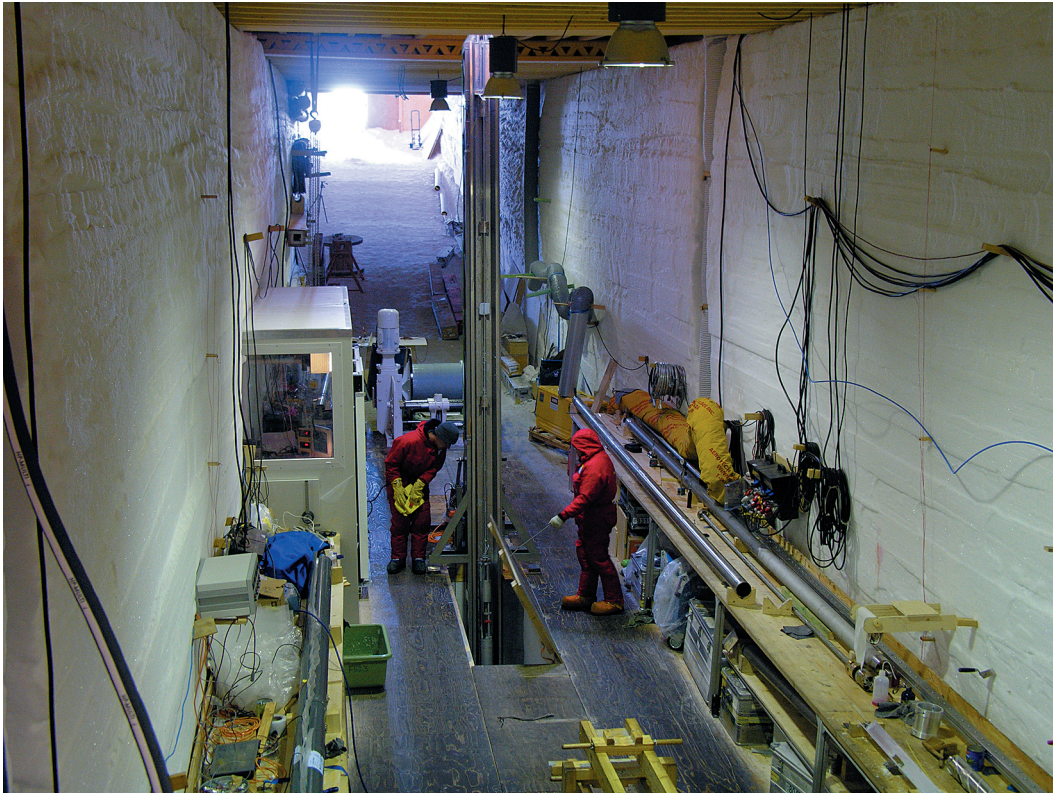
Fig. 16: View of the drill trench at Kohlen Station during drilling operation. The twelve metres long swivelling drill tower (the lower six metres are not visible) in the middle is standing upright and a new drill run just started. The last cover of the six metres deep inclined trench is getting closed. After the run it will be opened again to allow the tower to be tilted horizontally for taking out the core barrel. On the left, one can see the heated driller's hut with the control and steering device inside. At the beginning of a run the drill is steered via a remote control outside the hut. The winch with 3500 m of coaxial cable is visible behind the tower. The floor of the trench is covered by wood. Along the wall there are wooden tables on which the core barrel is placed for taking out the ice core. A special device (partly visible in the foreground center) with a small winch was constructed to pull out the core barrel from the outer tube, which some times got stuck very heavily. Air temperature inside the trench was around -30\text{ }^{\circ}\text{C} . (Photo H. Oerter, 12.12.2005).
