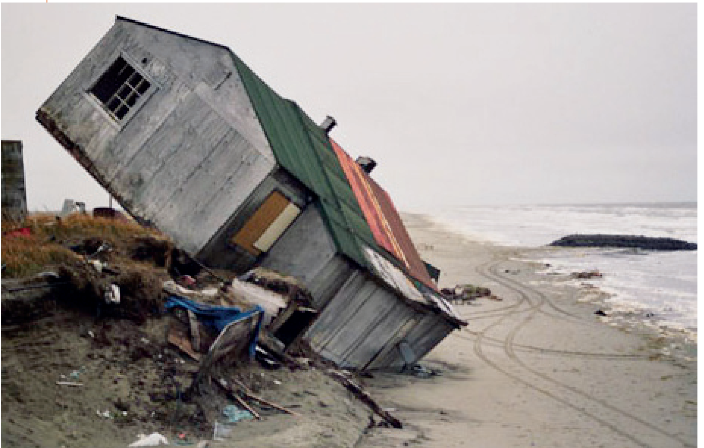
Figure 19: Coastal erosion of permafrost resulted in the complete destruction of this house in Shishmaref, Alaska.
