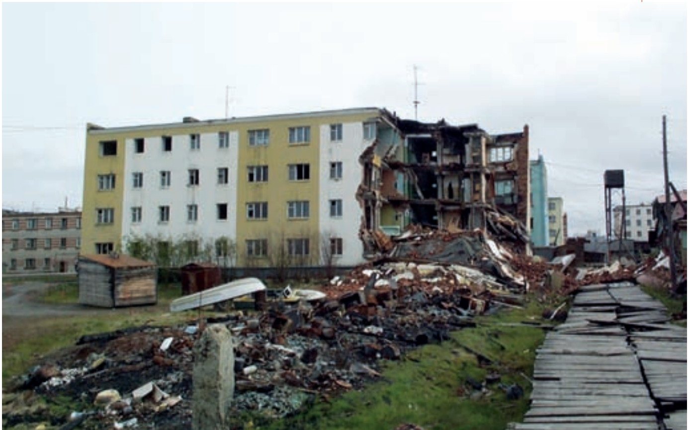
Figure 17: Uneven settling due to permafrost thaw destroyed this apartment building in Cherski, Siberia, which occurred only days after the appearance of the first cracks (photo: Vladimir Romanovsky).
