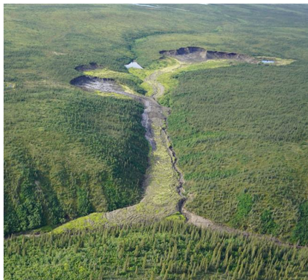
Figure 1. Large retrogressive thaw slump on Peel Plateau showing original disturbance feature (slump and headwall) which has grown to drain lake (rear right), vegetated upper debris tongue, upstream debris-dammed lake, secondary slumps on left side of valley, debris tongue and valley fill and valley-side erosion in foreground right.
