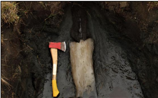
Figure 3: The ground has cracked during the winter 2017 (Foucault River).
