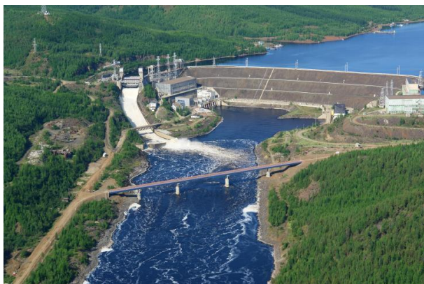
Figure 1. Vilyui Hydroelectric Station-1,2. General view.
