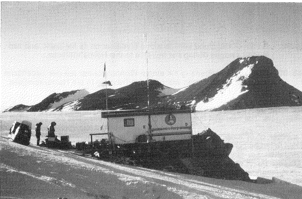
Fig. 39: The summer station SVEA in Scharffenbergbotnen. The station is constructed from two of the living containers carried on the Hägglunds. They were jacked up on their own legs and then welded together and after that anchored to the rocks.
