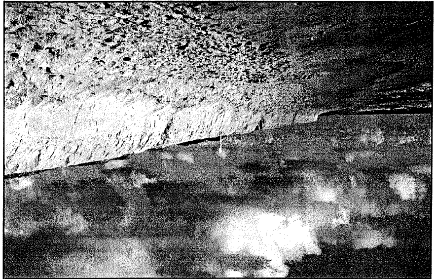
Fig. 9 Nourished sediment forms a new cliff on the beach of approximately 2.5 to 3 m depending on the volume of nourished material (island of Sylt, Germany).
