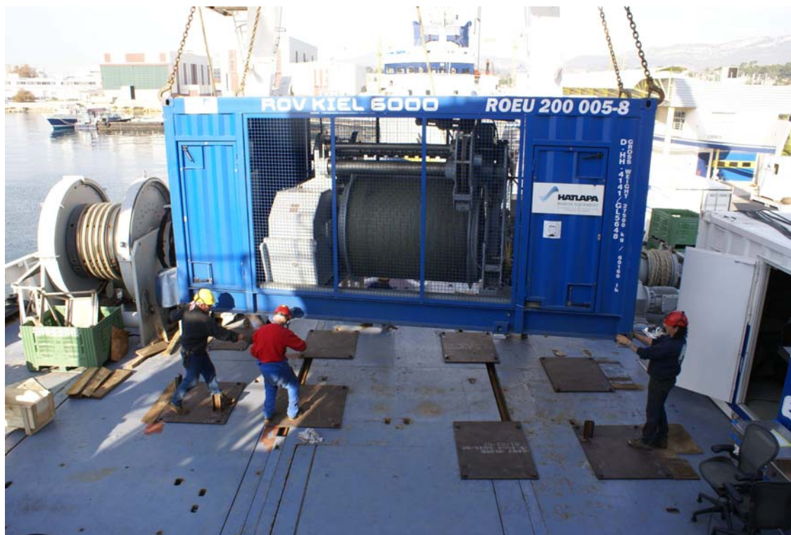
Fig. 1.4.10.2: Installation of the 28t winch with 6500 m of 19 mm umbilical for ROV KIEL 6000. Eight especially made base plates are used to fix the winch on deck (Foto: A. Massol, Ifremer).
