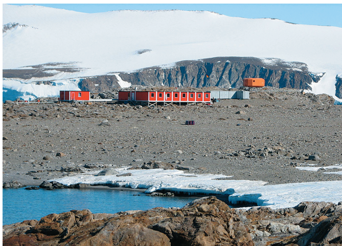
Fig. 5: The Gondwana Station of BGR at Terra Nova Bay. The main container assembly is flanked by the generator shed (left) and storage containers (right). The bright orange bivouac hut, which represented the first Gondwana station erected in 1983, had been moved from its original location to the present position when the new containerized station was built during austral summer 1988/89.
