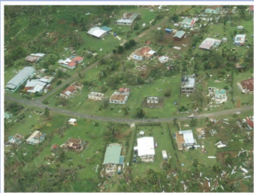
FIG. SB4.2. Widespread damage occurred in the village of Nikaupara on the island of Aitutaki in the Southern Cook Islands caused by Tropical Cyclone Pat in February 2010. (Photo Credit: Mr. Johnny Hosking in liaison with Air Rarotonga)
