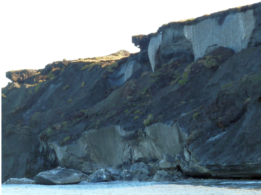
Fig. 20. Photograph of catastrophic collapse through undercutting, reflecting activation of TA during rising water level at the end of August 2011, when sea water comes in contact with permafrost in the level of thermo-niches. Under calm weather conditions the ground ice block decayed within two days.
