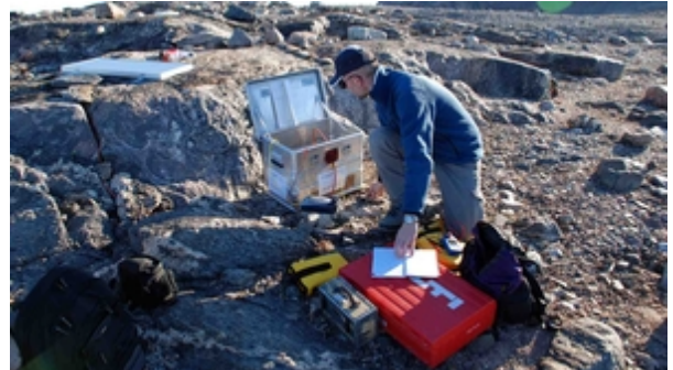
Installation of a geodetic station on Greenland (Photo: Ralf Rosenau)
