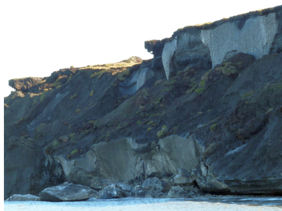
Figure 23. Photograph of catastrophic collapse through undercutting, reflecting activation of TA during the rising water level at the end of August 2011, when sea water comes in contact with permafrost at the level of thermo-niches. Under calm weather conditions the ground ice block decayed within 2 days.
