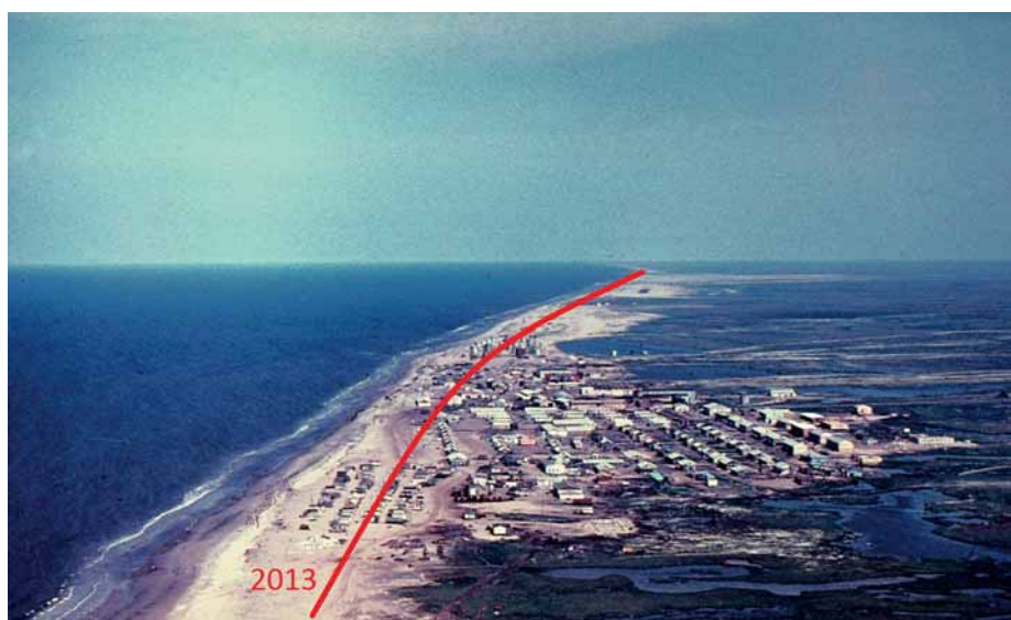
Fig. 11. Aerial photo of the Varandey settlement at 1985; coastline of 2013
