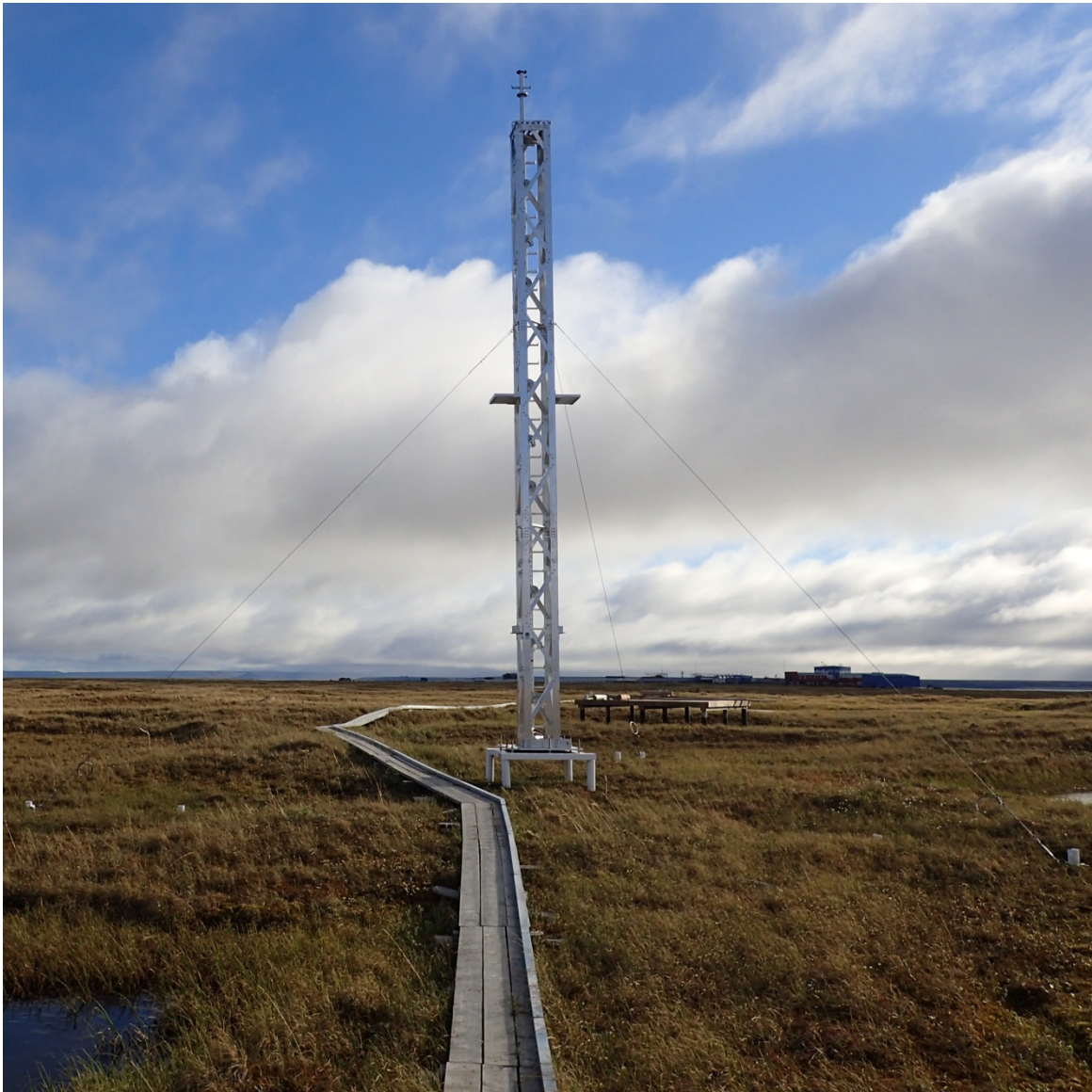
Figure 2.3.-2: New ACROSS research infrastructure: wooden boardwalk, 10 m tower, (SaTower2016). The wooden platform will be used as base for the climate controlled container. Samoylov research station is visible in the background.
