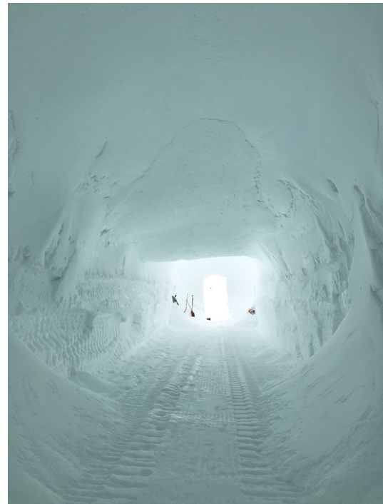
Fig. 4.19.4: Looking west to the entrance. The ceiling is designed as a vault at the top of the picture, but then drops significantly.
