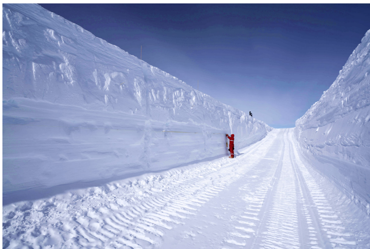
Fig. 5.5.2: The excavated 50 m long and 4 m deep T4M-trench
